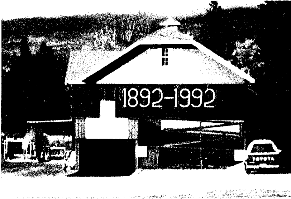
East side of building with Fire Hall. "1892-1992" sign celebrates Silverton's 100 years. SHS A006-001-0407
