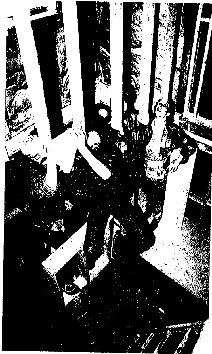
STRAINING FOR THE SAKE OF ART — Some odd expressions were the result this week as four workers renovating the Silverton Elementary School put beams into place. The four are converting the 1919 building from a two-room schoolhouse into a visual and performing arts centre to serve the upper Slocan Valley. From left to right the men are Bill Emmett, Phil Milbourn, Bob Potumbo and the "foreman", Joel Harris. Michael Hartley photo
